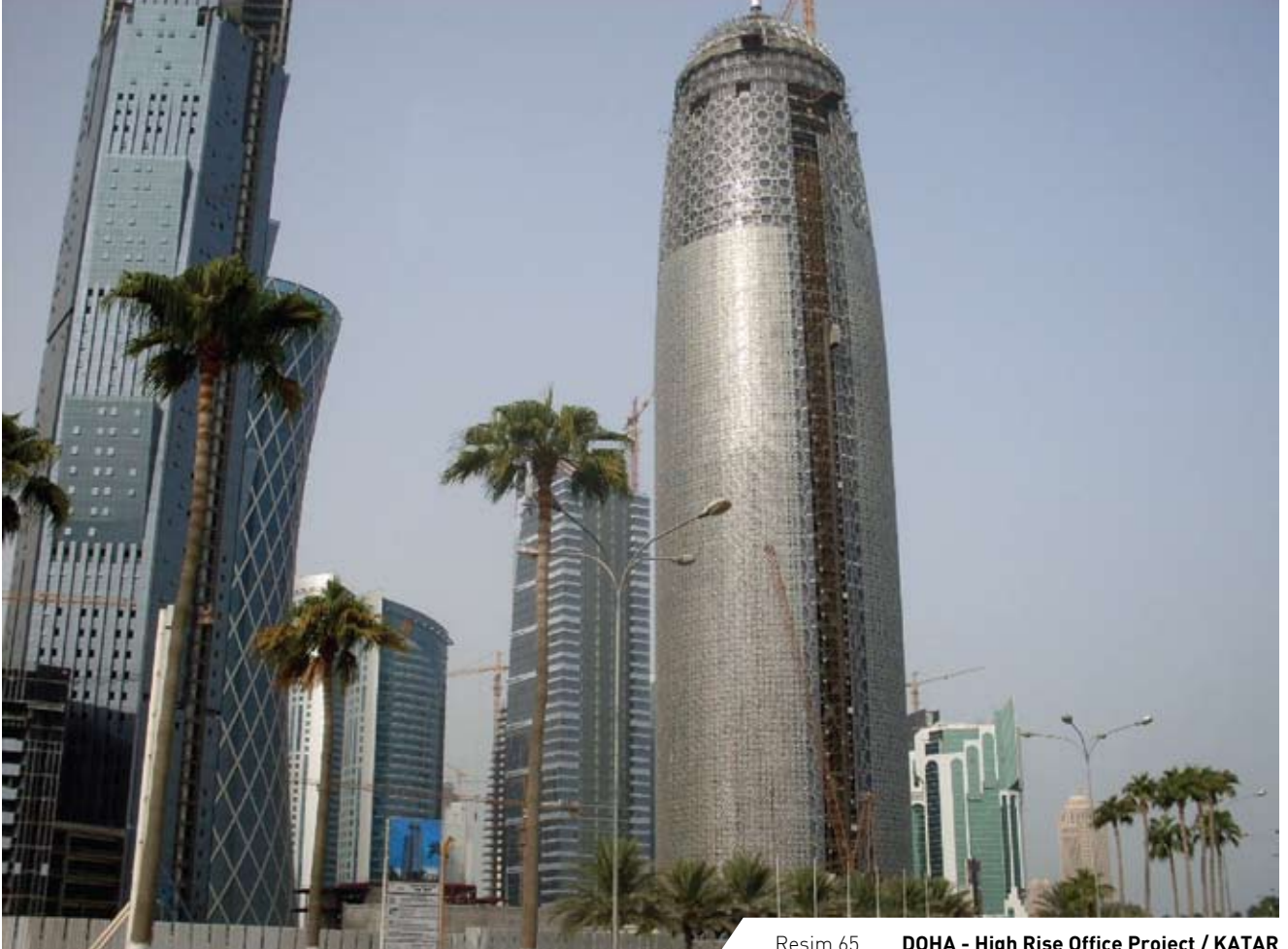
Resim 65 DOHA - High Rise Office Project / KATAR
